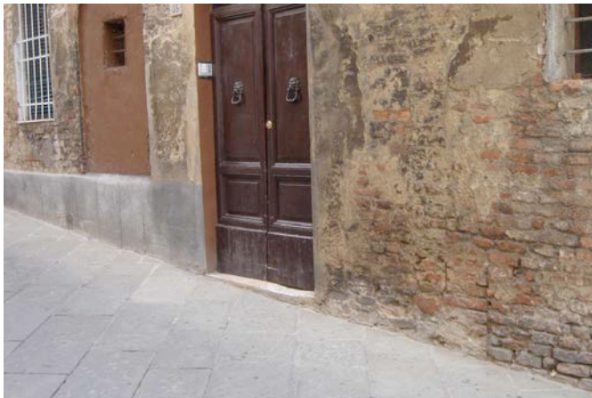
Photograph 4: New sacrificial layer in Firenze, Italy
