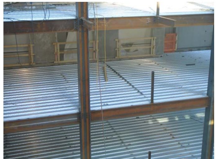
Photograph 6: Fluted Steel Deck
