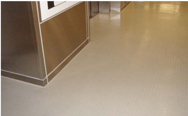
Photograph 8: Vinyl Composition Flooring
