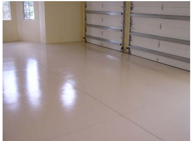
Photograph 7: Epoxy Coatings
