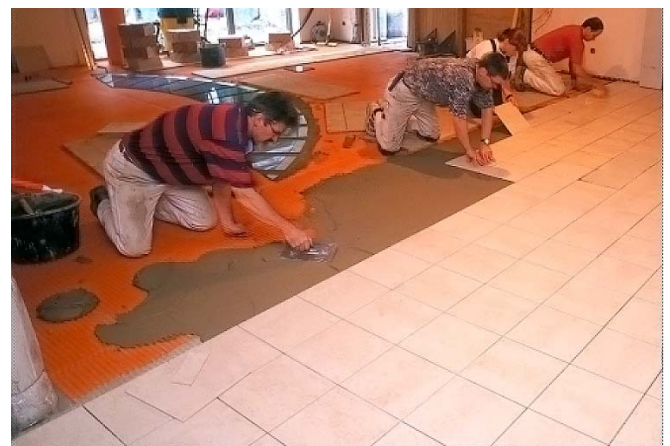
Photograph 11: Tile Installation
