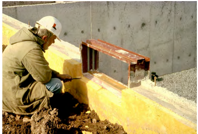
Photograph 2: Mastic Water Control Layer (above left) —It was not practical to install building paper over a masonry “back-up” wall. You can’t staple it, you can’t nail it. What did we have available at first? We used mastics – basically below grade waterproofing - and then “peel and stick” membranes were developed. Today we have fluid applied and spray applied water control layers to go over masonry “back-up” walls. Photograph 3: Below Grade Draining Insulation (above right) —Fiberglass. I got my first real education in draining insulations in the late 1970’s doing exterior foundation insulation using fiberglass roofing insulation. Yes, that is Professor John Timusk on a job site in Brampton, Ontario in 1979, trimming the exterior basement draining insulation.
