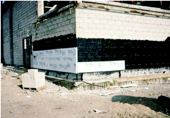
Photograph 2: Mastic Water Control Layer (above left) —It was not practical to install building paper over a masonry “back-up” wall. You can’t staple it, you can’t nail it. What did we have available at first? We used mastics – basically below grade waterproofing - and then “peel and stick” membranes were developed. Today we have fluid applied and spray applied water control layers to go over masonry “back-up” walls. Photograph 3: Below Grade Draining Insulation (above right) —Fiberglass. I got my first real education in draining insulations in the late 1970’s doing exterior foundation insulation using fiberglass roofing insulation. Yes, that is Professor John Timusk on a job site in Brampton, Ontario in 1979, trimming the exterior basement draining insulation.
