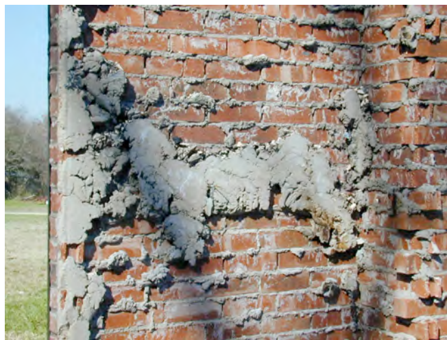
Photograph 1: Mortar Droppings —The gap was the rain control thing in the original cavity walls. And the key to the gap was to keep the mortar out of the gap. The bigger the gap, the easier it was to keep the mortar out of it. A 2-inch gap worked great.
