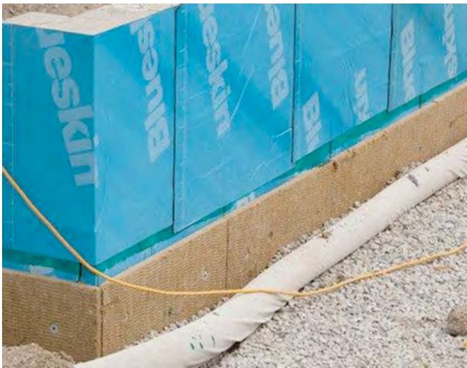
Photograph 4: Below Grade Draining Insulation (above left) —Rock Wool/Stone Wool. Today, rock wool (“stone wool”) is commonly used as a draining insulation below grade on the exterior of foundations. Photograph 5: Above Grade Draining Insulation (above right) —Rock Wool/Stone Wool. If you can use rock wool/stone wool below grade you certainly can use it above grade on the exterior of a water control layer.
