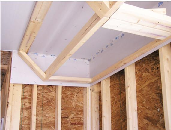
**Photograph 3 (at left): Bulkhead Framing** – Moving the ductwork into conditioned space typically requires bulkheads and soffits that are airtight.
