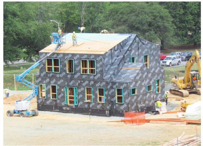
Photograph 1: Ultra Tight House – Advanced frame house sealed with a fully adhered exterior air control layer installed over structural sheathing yields an enclosure with a leakage rate less than 0.5 ach@50 Pa as tested under pressurization or depressurization.
