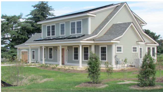
Photograph 3: Completed Ultra Tight House – Looks like any other house, just tight and ventilated right. Balanced fully ducted heat recovery ventilator with sealed combustion appliances and powered make-up air when air consuming appliances are used. OK, it doesn't quite look like any other house because of the PV array and solar thermal stuff. This is the NIST Zero Energy Demonstration House in Gaithersburg, MD.
