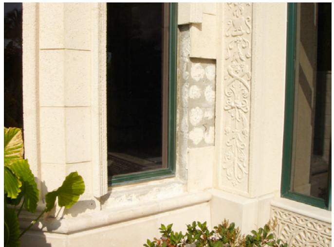
Photograph 6: Perched Water (below) —The "blobs" are too big, and there are too many of them, and they are too close together and lead to perched water.
