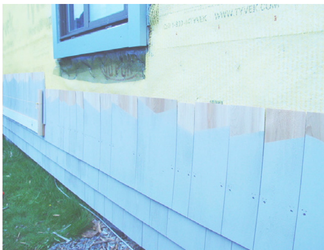
Photograph 2: Gap Behind Siding and Trim (left) —With wood and fiber cement siding and trim you need to install the siding and trim over a small gap to control hydrostatic pressure. This gap can be as small as a 1/4-inch and the spacer can be a strip of thin foam.
